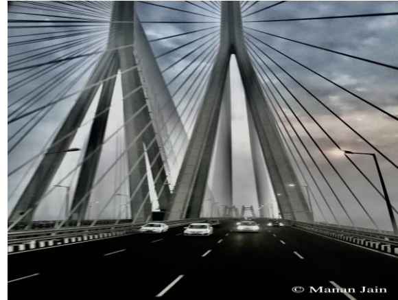
Fig 5.18 Main cable-stayed span
