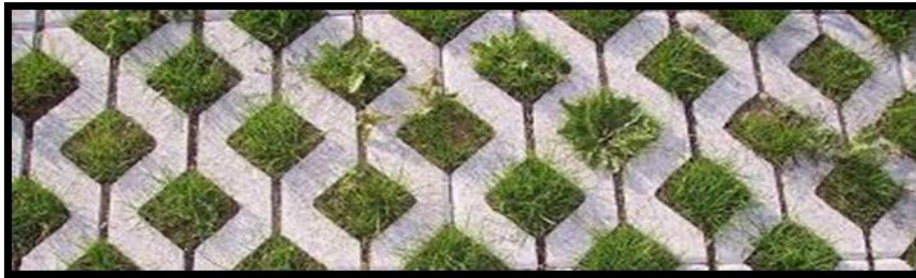
Fig 5.4 Grass cell paving.
